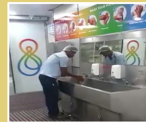
Sliding door opens based on activation of pressure switch due to flow of water during hand wash
